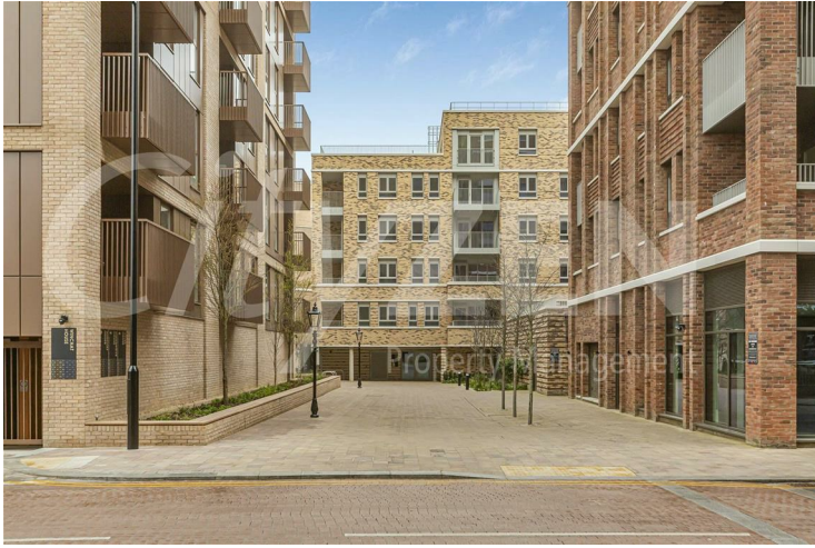
ENTRANCE TO WINCHAT HOUSE
